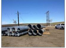
The Worden tap is a double-circuit 115kV transmission line to a new substation. The line is all self-supporting steel poles in poor soils with a full-length static and provisions for two fiber optic cables. The two primary challenges on this project were landowners with changing requests very late in the design process, and the poor soils necessitating a challenging footing design to support the double-circuit transmission.
